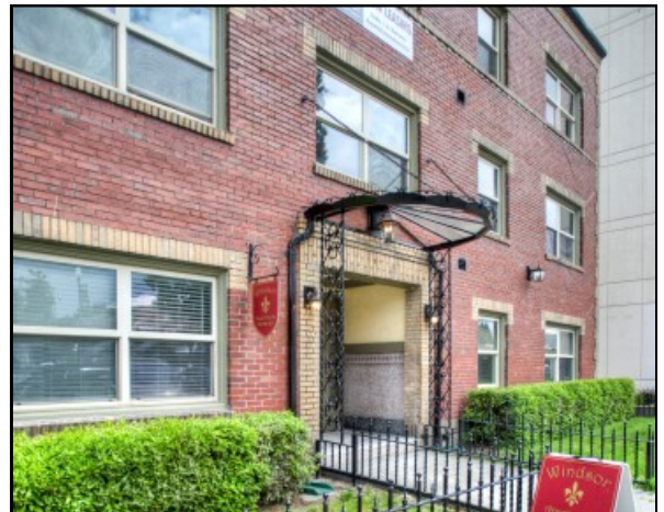
The Windsor now available. Total rehab.
